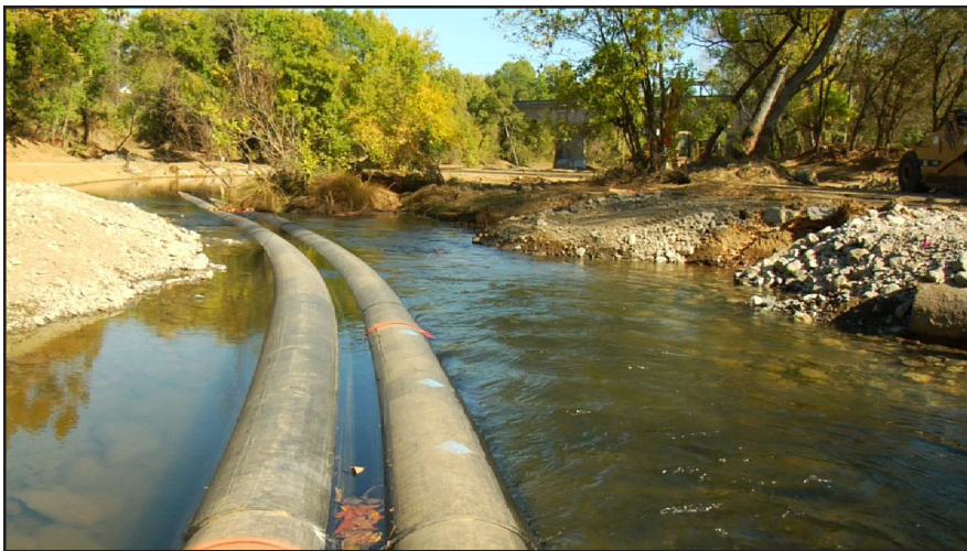
Re-wetting the creek bed with pipes. Neil Crossing
