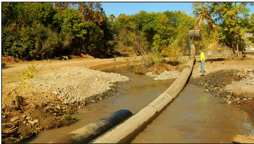
Removing water conveyance pipes
